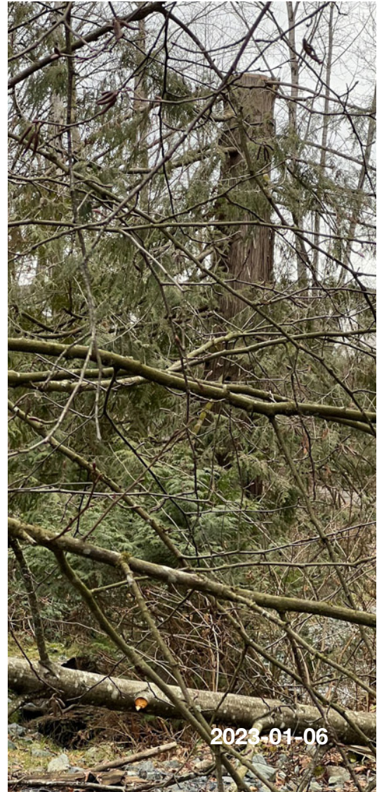
The shambles at Bridge 5
